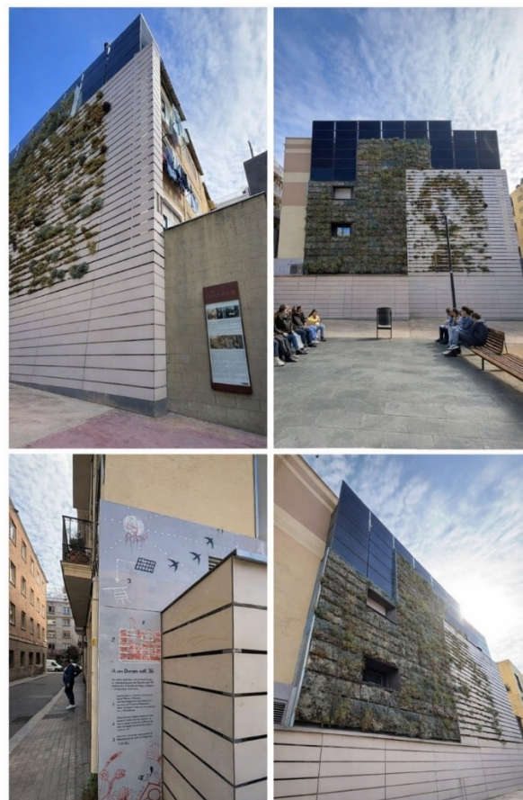
Figure 13. Biodiversity-oriented façade system in Barcelona integrating vertical vegetation and photovoltaic panels to provide habitat for urban species while generating energy (author's archive, April 16, 2026).
